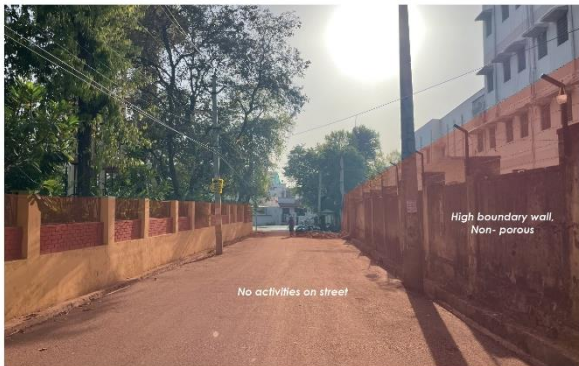
Figure 26 Absence of footpath, benches and active facade, no eyes on street
