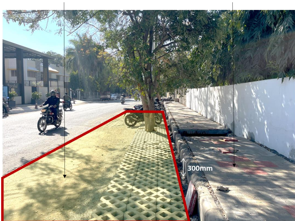
Figure 27: Existing condition of Saheli Marg. Source: (Author, 2022)
