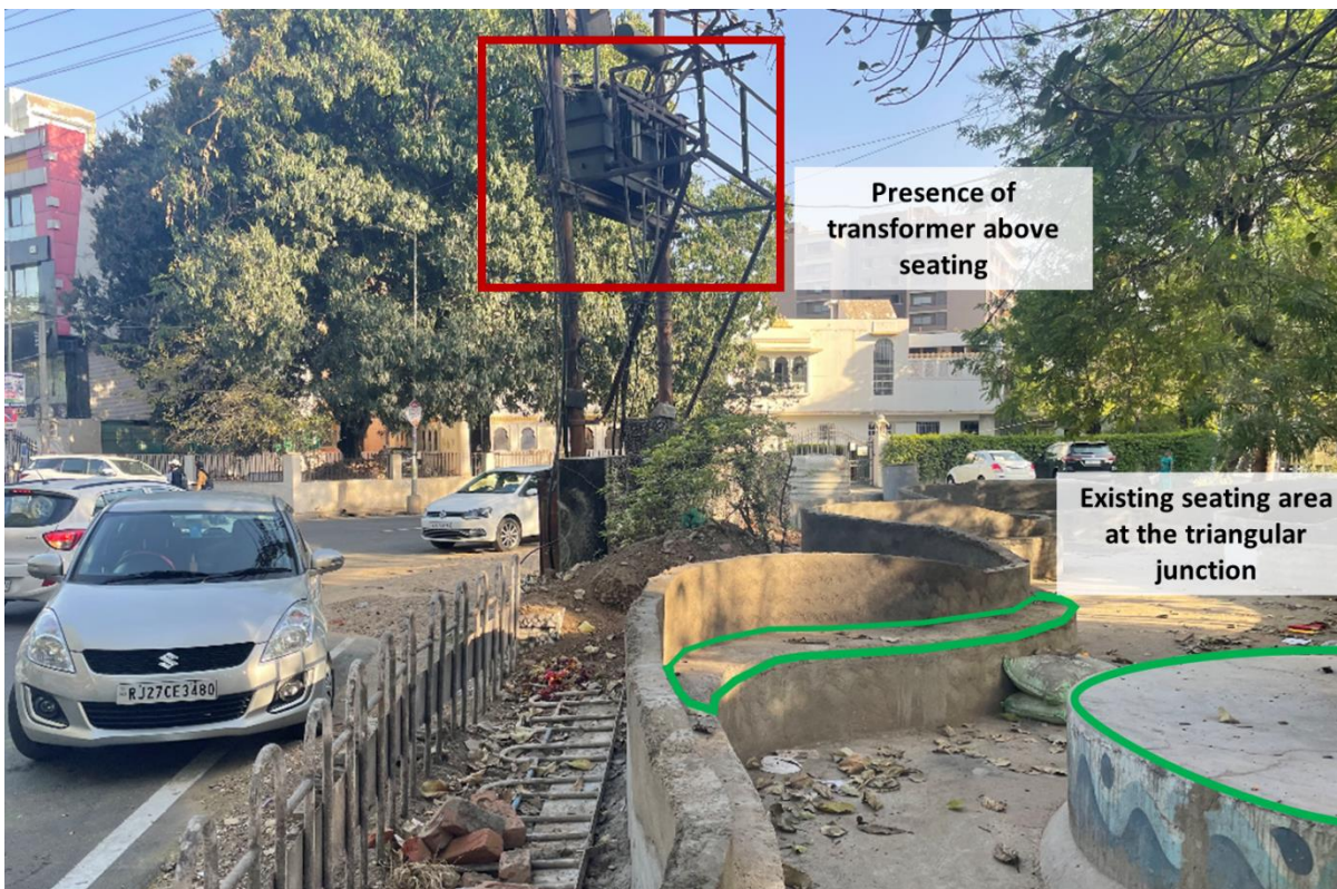
Figure 26: The transformer placed above seating risks the safety of caregivers. There is lack of barricade to safeguard children from the poles. Source: (Author, 2022)
