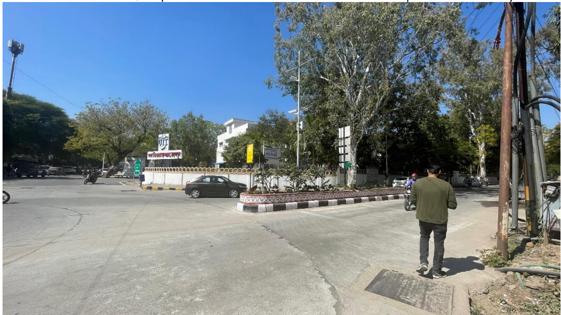
Figure 29: UIT Circle after improvements. Source: (Author, 2022)
