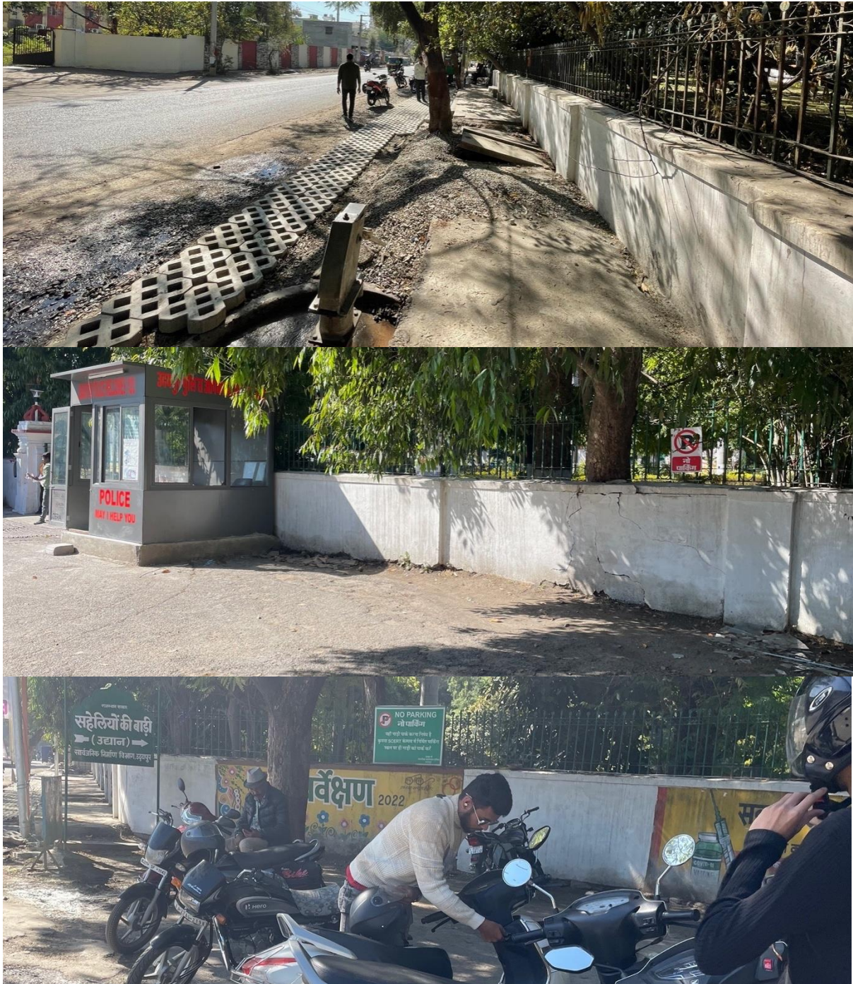
Figure 64: Dead Boundary walls near Saheliyon Ki Bari. Source: (Author, 2022)
