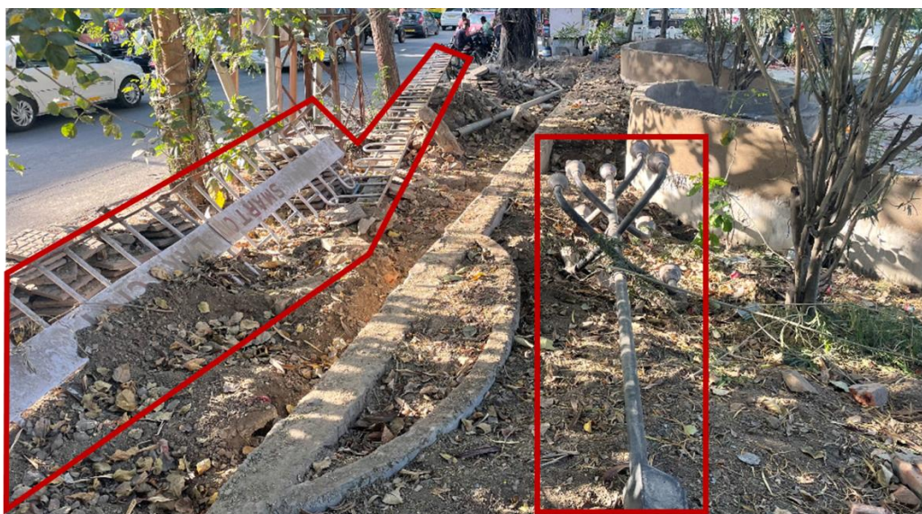
Figure 24: Poorly maintained potential public space and dilapidated infrastructure at Saheli Marg triangular junction, Source: (Author, 2022)
