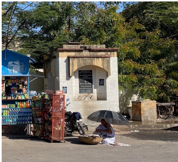
Figure 67: Drinking water facility existing at Sahilyon Ki Bari Junction. Source: (Author, 2022)
