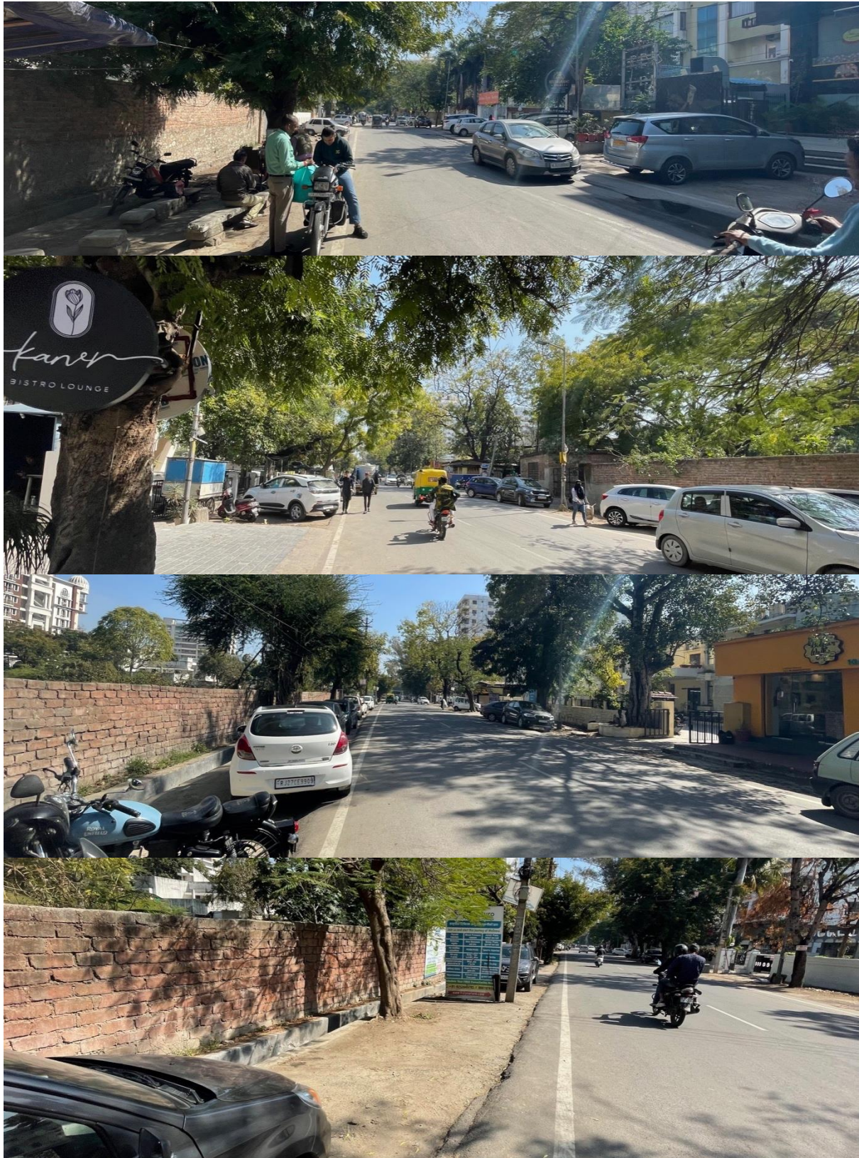
Figure 65: Sections of Dead Boundary walls along Big Bazar Road. Source: (Author, 2022)
