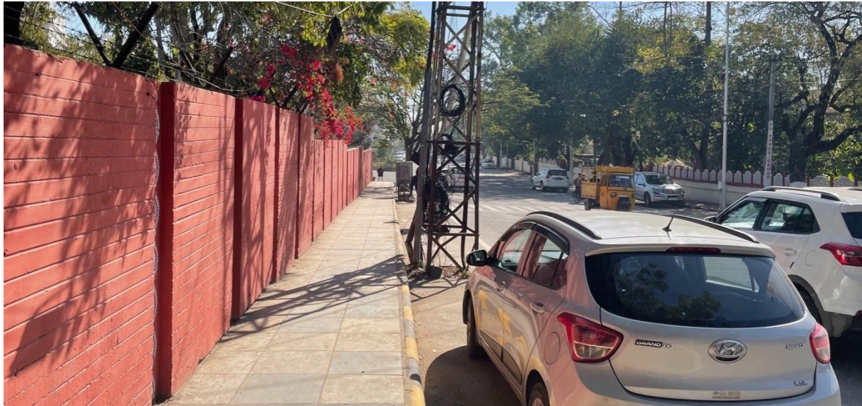
Figure 66 Existing dead boundary wall near Fatehpura Junction. Source: (Author, 2022)
