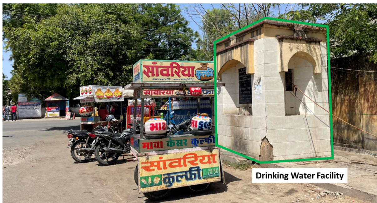
Figure 18: Existing drinking water facility supports ITC infrastructure, Source: (Author, 2022)
