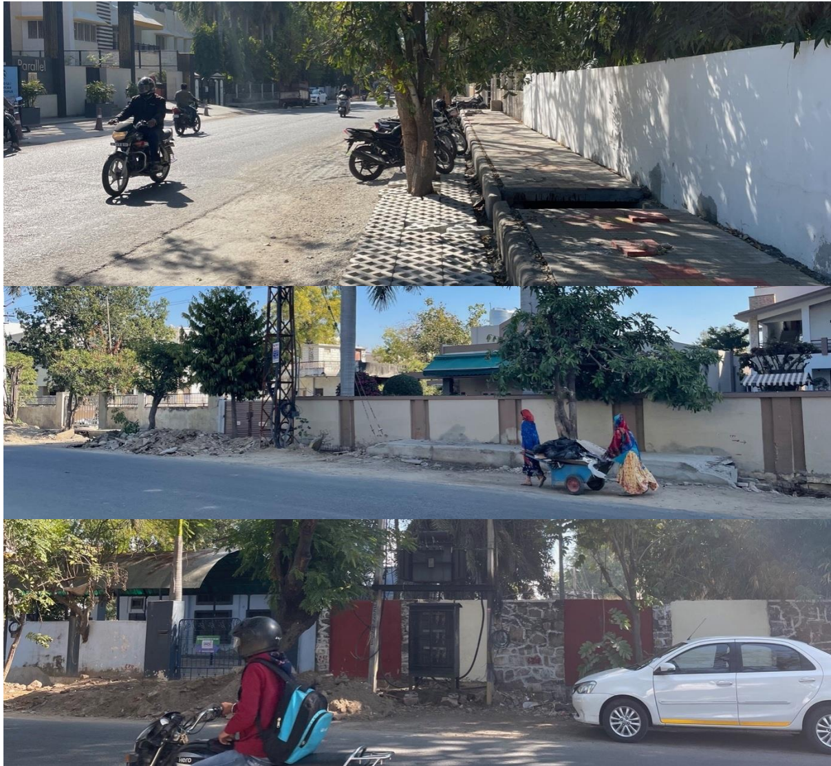
Figure 63: Dead Boundary walls along Saheli Marg. Source: (Author, 2022)
