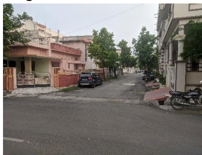
Figure 26 Absence of sidewalks near grocery stores, open drains & ramps
