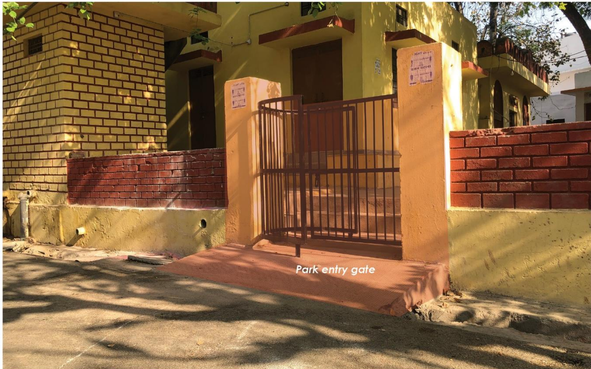
Figure 42 Hanuman Park entrance is an issue for strollers to access
