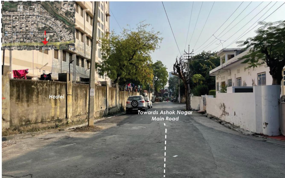
Figure 9 The access road leading towards (anchor institute) Hanuman Park, and Ashok Nagar main road requires ITC's friendly designs on the intersection for engaging young children
