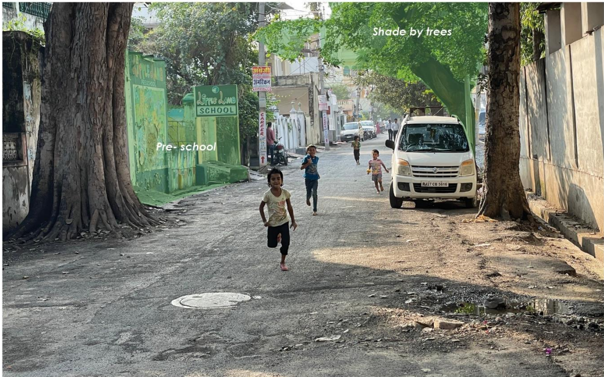
Figure 34 Trees act as natural shading elements on the stretch, adequate light poles, and pre-school available
