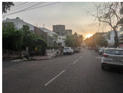
Figure 28 Open drains and encroachment on street by ramps and parked vehicles
