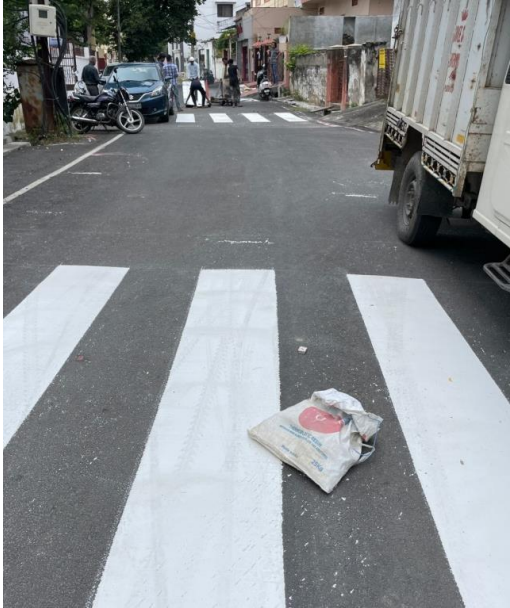
Work in Progress – Usage of thermoplastic paints for road markings
