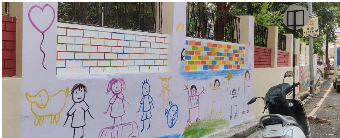
Paintings - completed work on the boundary walls of the Park
