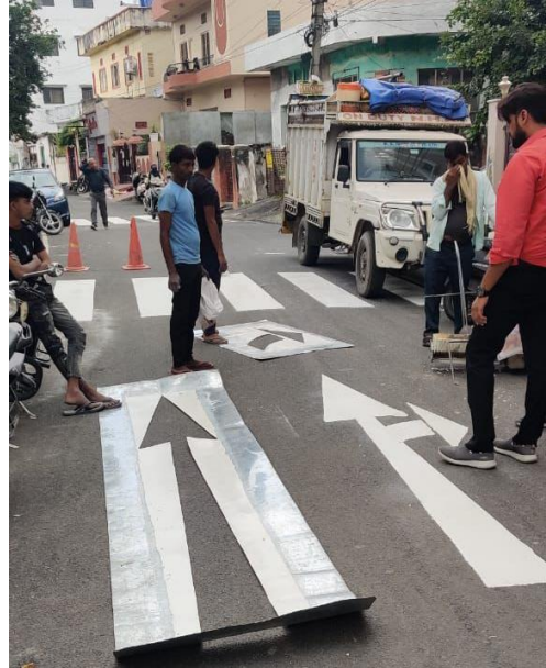
Work in Progress – Usage of thermoplastic paints for road markings
