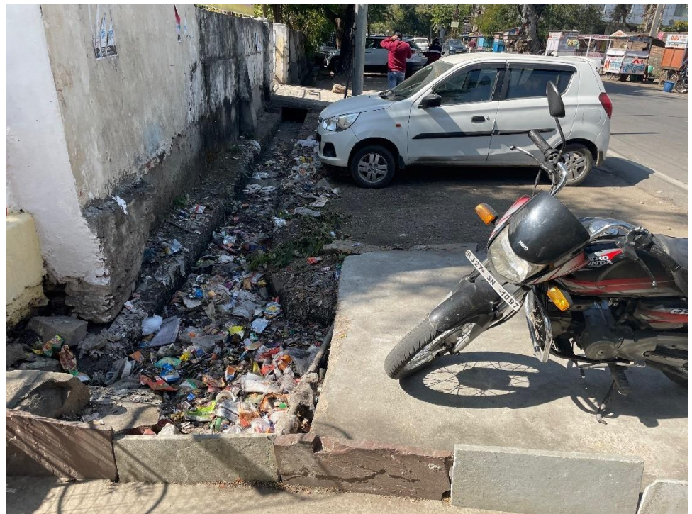
Portion of Storm water drain near Sukhadiya Circle
