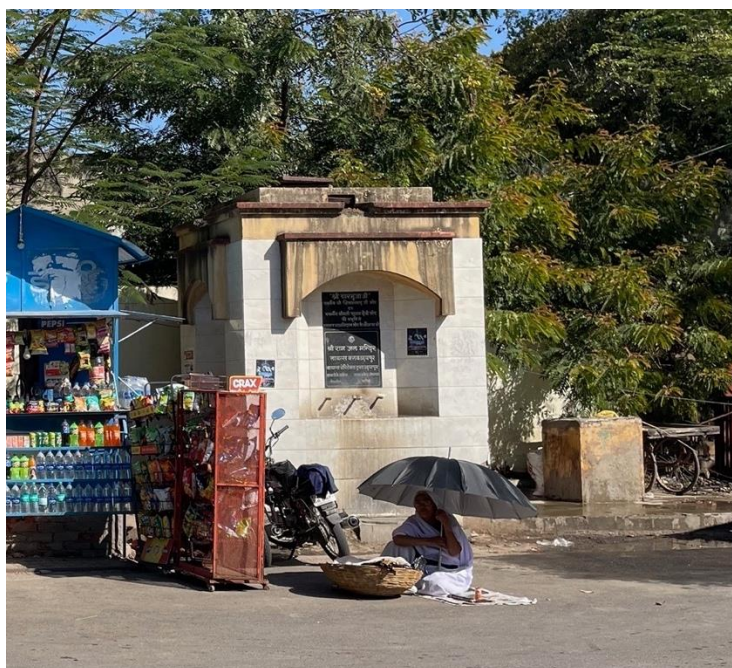
Drinking water facility existing at Sahilyon Ki Bari Junction
