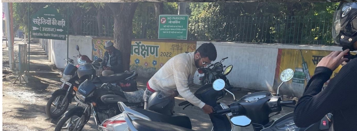
Dead Boundary walls near Saheliyon Ki Bari.
